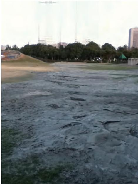
Figure 2.1-25 Liquefaction in Makuhari Kaihin Park (photo taken on March 18)
