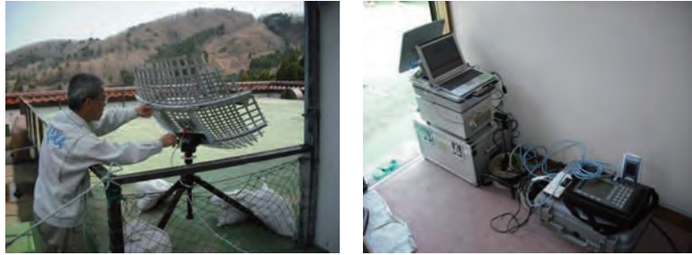
Figure 2.2-26 Communication equipment and other devices installed (left: antenna; right: equipment and supplies)
