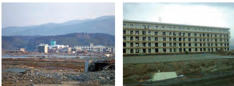
Figure 2.2-21 Tsunami damage (near Rikuzentakata City)
