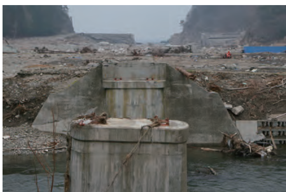
Figure 2.1-67 Settai district, Miyako City, Iwate The site of a village and a bridge claimed by the tsunami
