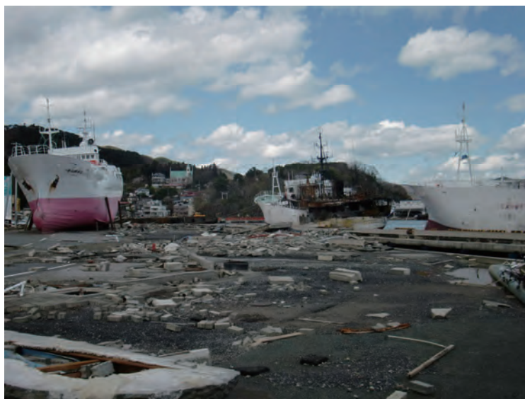
Figure 2.1-69 Harbor affected by subsidence in Kesennuma City, Miyagi
