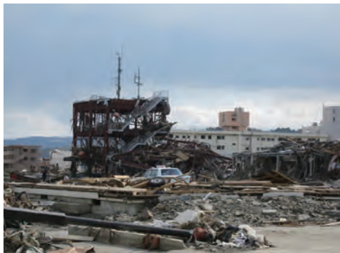
Figure 2.1-70 Minamisanriku Town, Miyagi Damaged town hall (Photo courtesy of Asia Air Survey Co., Ltd.)
