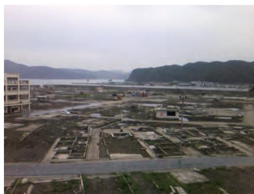
Figure 2.1-68 Taro district, Miyako City, Iwate Damage to an area with tsunami barriers
