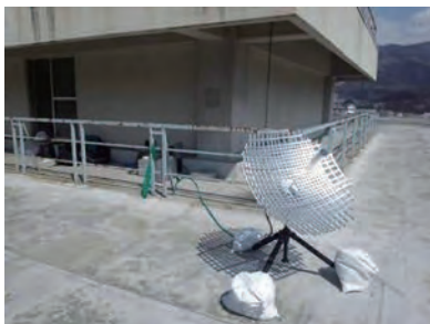
Figure 2.2-18 Communication equipment installed (left: 90 cm \phi portable antenna; center: portable communication terminal equipment; right: portable generators)
