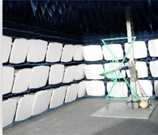
EMC Anechoic Chamber
